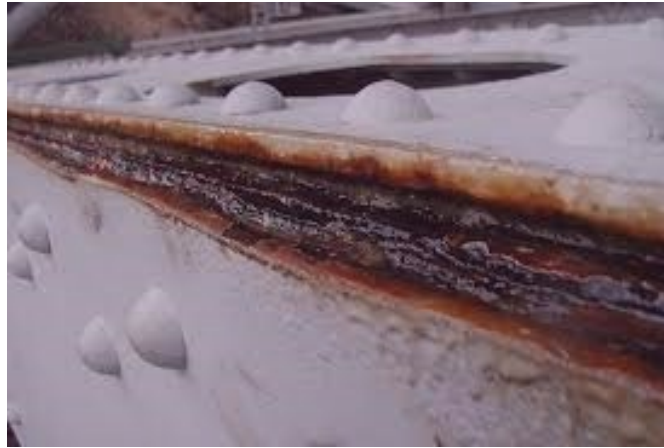
Figure 1.7: Crevice Corrosion
